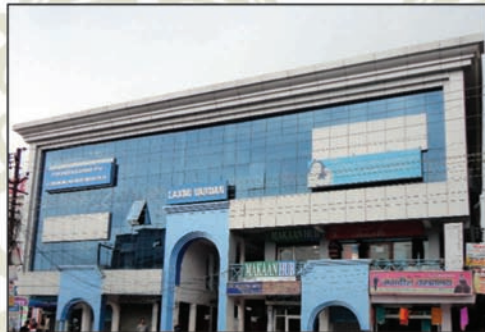
Laxmi Vardhan Complex, Patrakar Puram Crossing, Gomti Nagar
